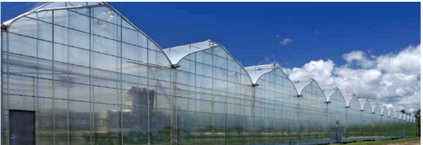
8 mm, double wall polycarbonate panels: this rigid covering offers excellent durability and good insulation.
